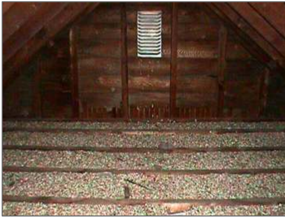
Vermiculite attic insulation
