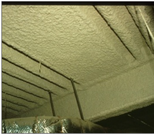
Cementitious sprayed fireproofing
