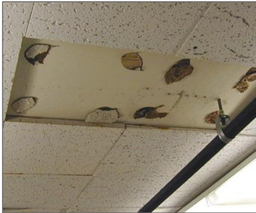
Glued on (laminated) ceiling tiles
