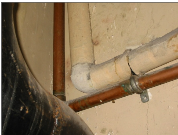
Parging cement on pipe fitting
