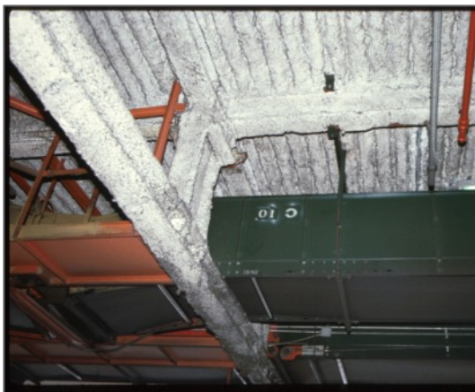
Fibrous sprayed fireproofing
