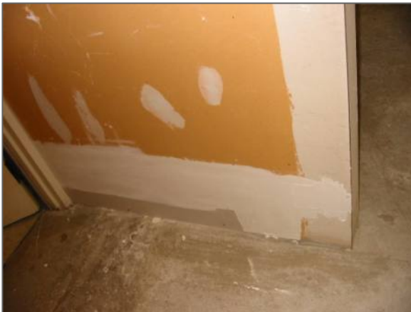
Drywall joint compound on drywall
