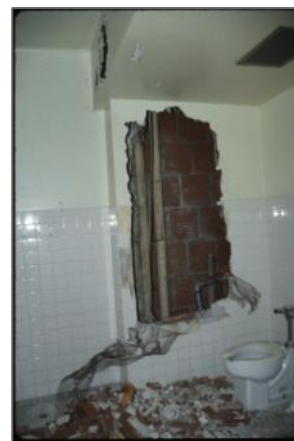
Plaster on speed tile
