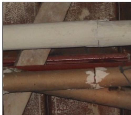
Parging cement on sweatwrap and Aircell
