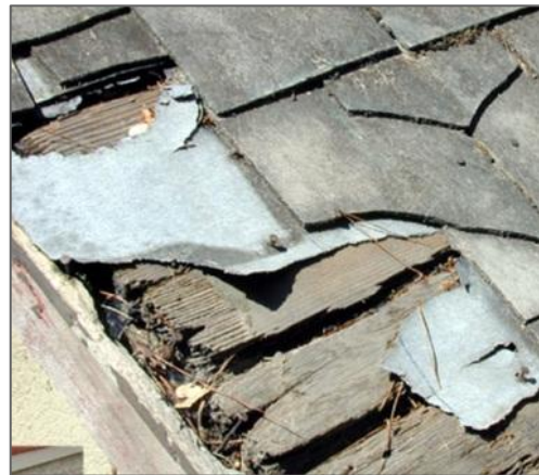
Building paper under roof tiles
