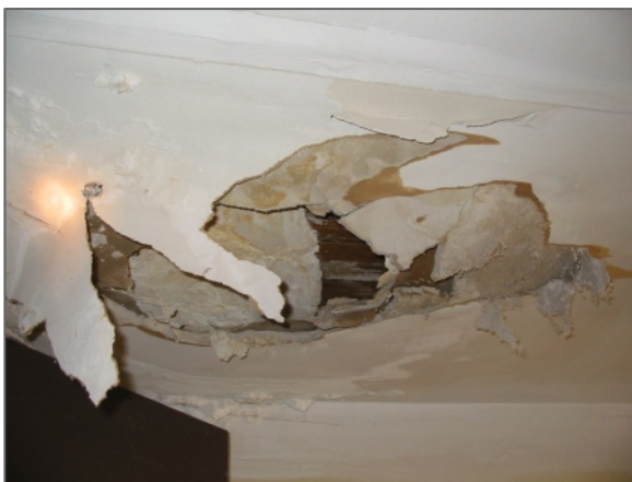
Plaster on wood lath
