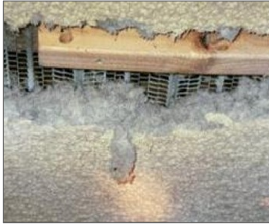
Sprayed limpet texture ceiling on lath
