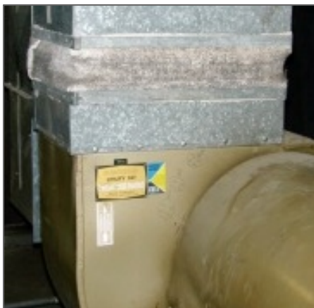
Textile Vibration Damper/Duct Connector
