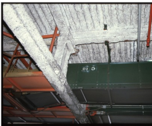
Fibrous sprayed fireproofing
