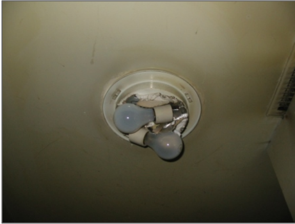
Paper heat shield on incandescent fixture
