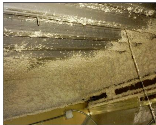
Fibrous sprayed fireproofing (beam only)
