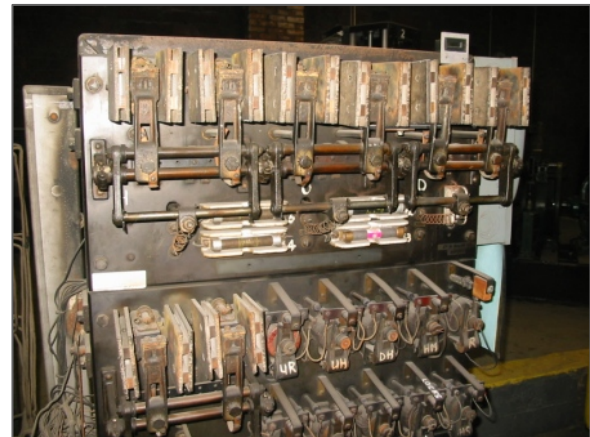
Transite Blocks in Elevator Switchgear
