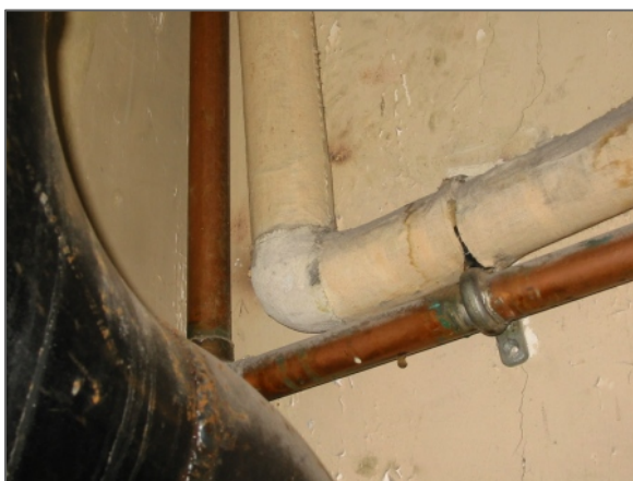
Parging cement on pipe fitting
