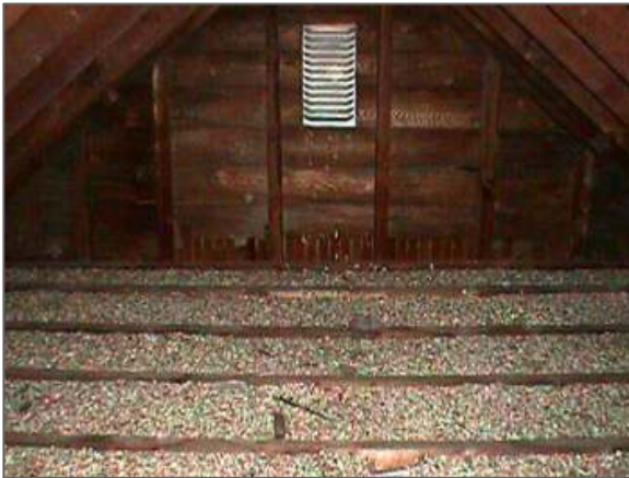
Vermiculite attic insulation
