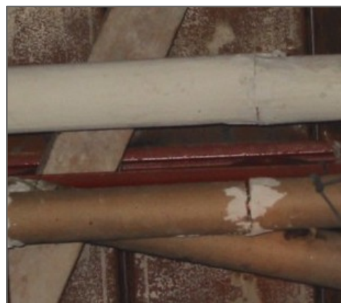
Parging cement on sweatwrap and Aircell
