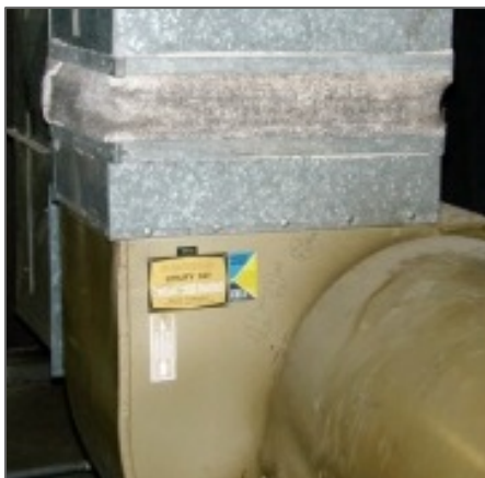
Textile Vibration Damper/Duct Connector
