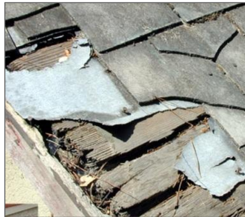
Building paper under roof tiles
