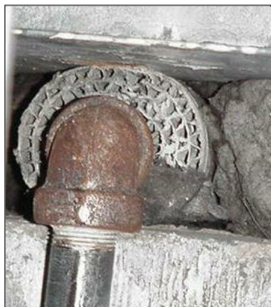
Aircell insulation (corrugated paper)
