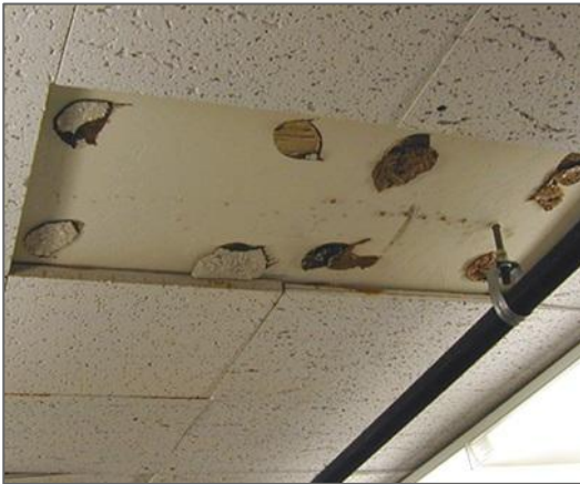
Glued on (laminated) ceiling tiles
