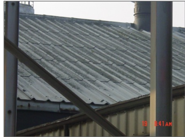
Corrugated Transite Siding/Roofing
