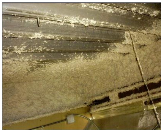
Fibrous sprayed fireproofing (beam only)
