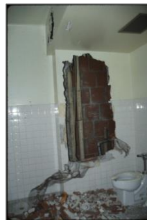
Plaster on speed tile
