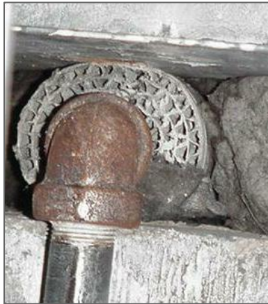
Aircell insulation (corrugated paper)
