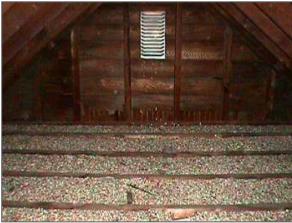
Vermiculite attic insulation
