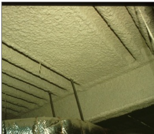
Cementitious sprayed fireproofing
