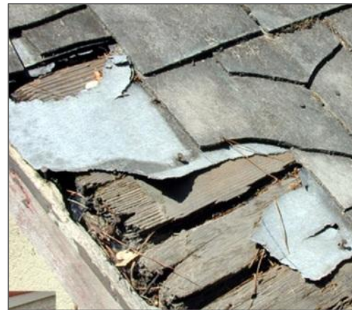
Building paper under roof tiles
