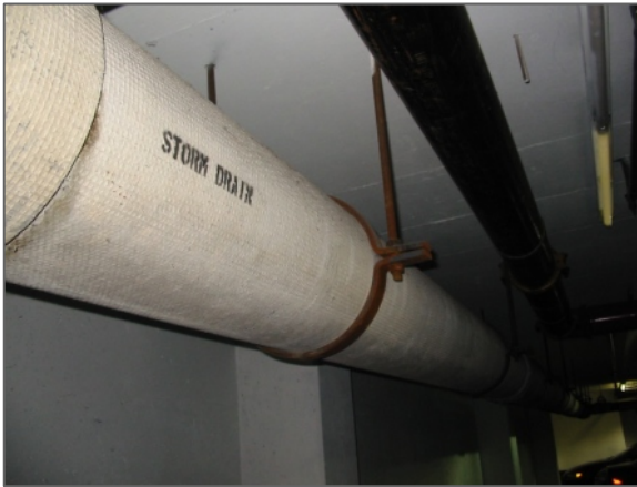
Transite Drain Pipe
