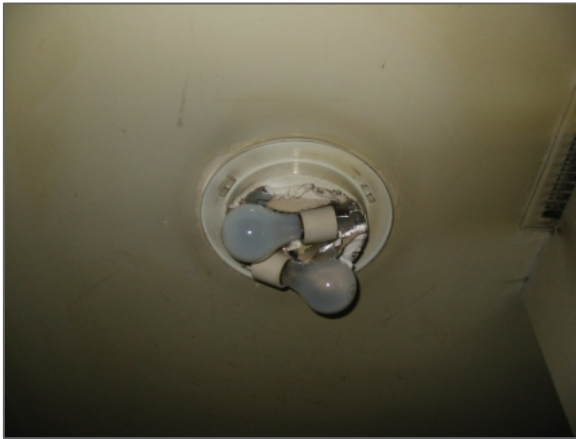
Paper heat shield on incandescent fixture
