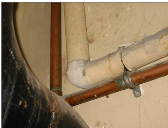
Parging cement on pipe fitting
