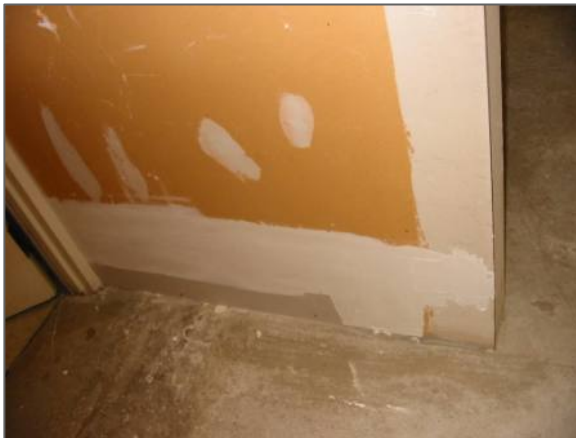
Drywall joint compound on drywall
