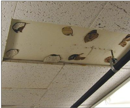
Glued on (laminated) ceiling tiles
