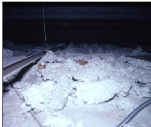
Debris from fireproofing on top of ceiling
