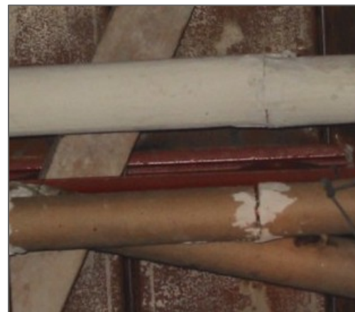
Parging cement on sweatwrap and Aircell
