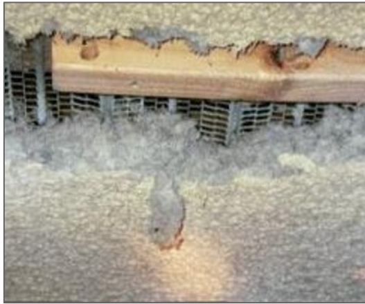
Sprayed limpet texture ceiling on lath
