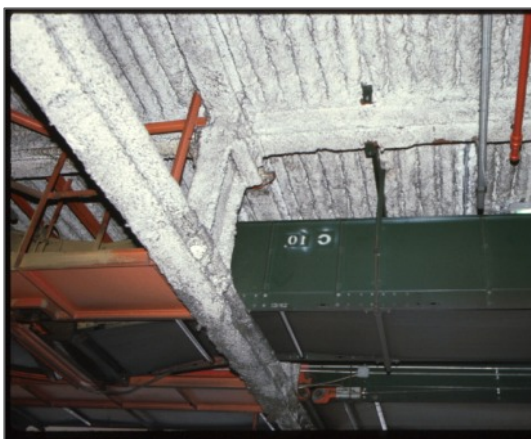
Fibrous sprayed fireproofing
