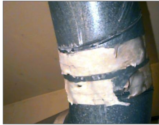
Paper on seams of duct
