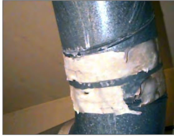
Paper on seams of duct
