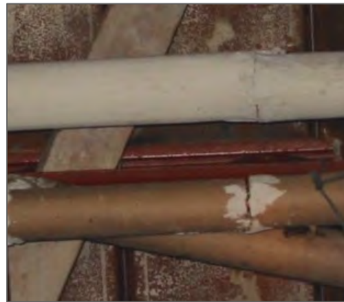
Parging cement on sweatwrap and Aircell
