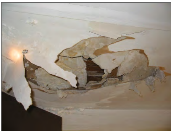
Plaster on wood lath
