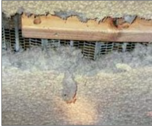
Sprayed limpet texture ceiling on lath
