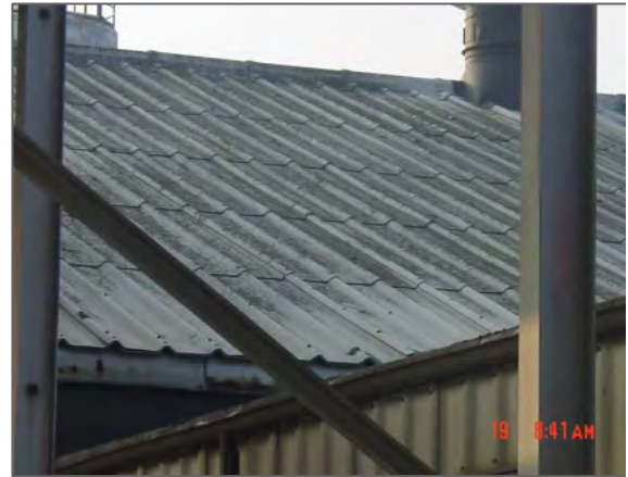
Corrugated Transite Siding/Roofing
