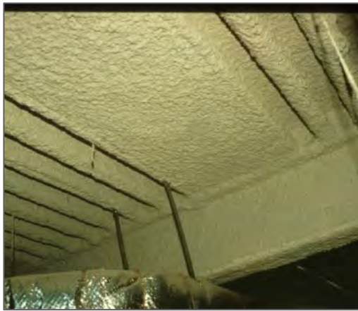
Cementitious sprayed fireproofing
