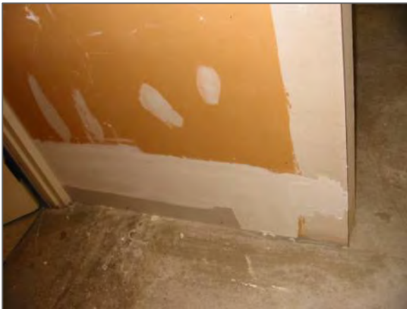
Drywall joint compound on drywall
