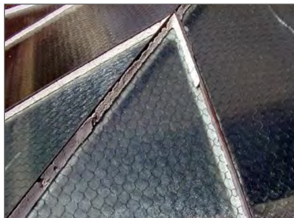
Caulking at Glazing
