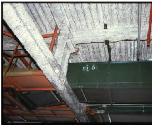
Fibrous sprayed fireproofing
