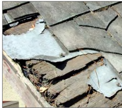
Building paper under roof tiles
