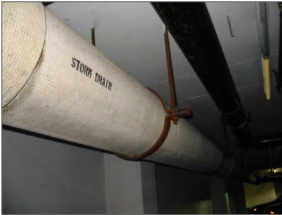
Transite Drain Pipe
