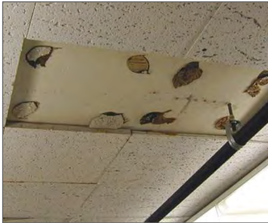
Glued on (laminated) ceiling tiles
