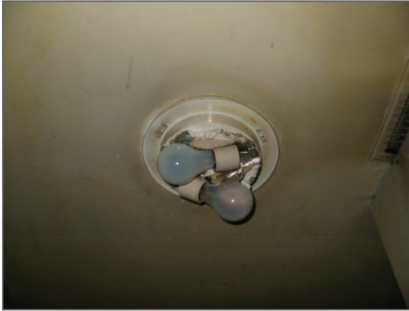
Paper heat shield on incandescent fixture
