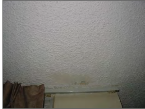
Texture coat ceiling
