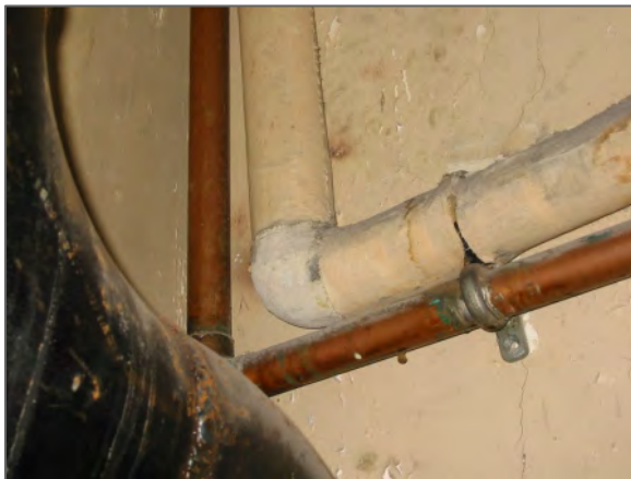
Parging cement on pipe fitting
