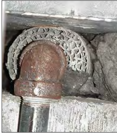
Aircell insulation (corrugated paper)
