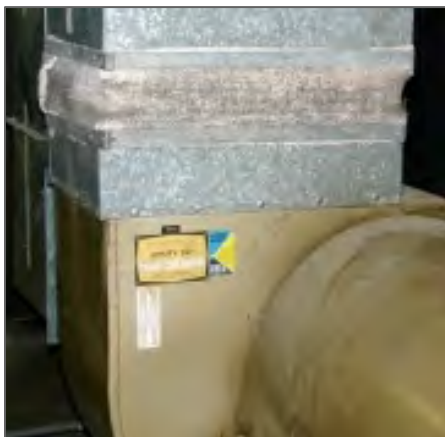
Textile Vibration Damper/Duct Connector
