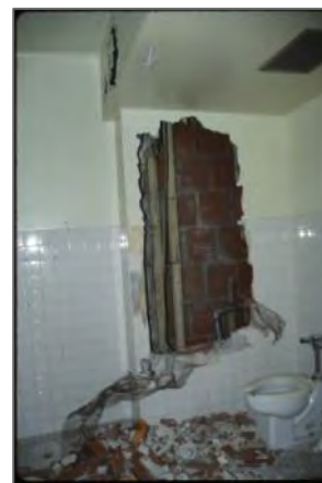
Plaster on speed tile
