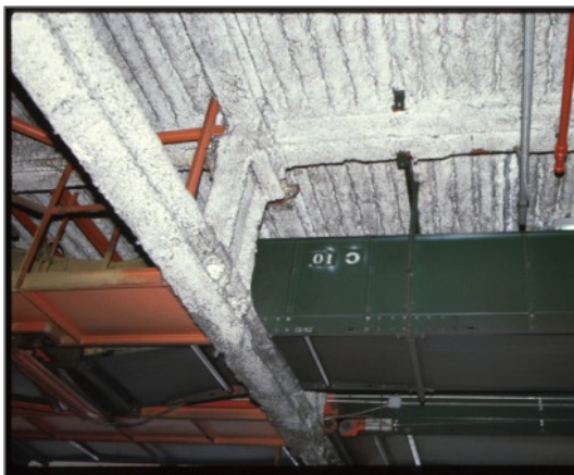
Fibrous sprayed fireproofing
