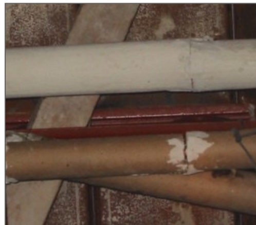
Parging cement on sweatwrap and Aircell
