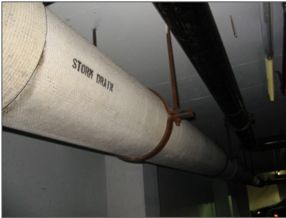
Transite Drain Pipe
