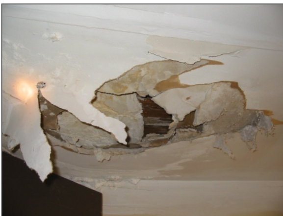
Plaster on wood lath
