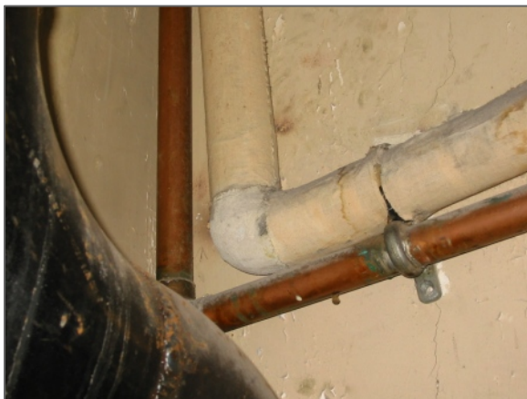
Parging cement on pipe fitting
