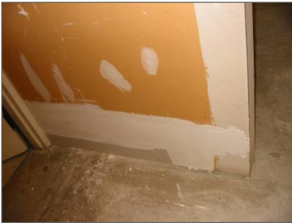
Drywall joint compound on drywall
