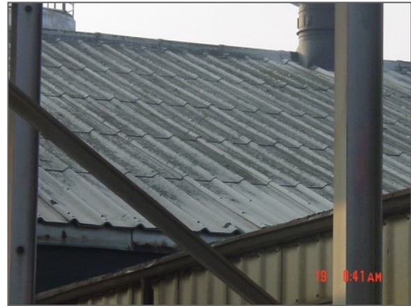
Corrugated Transite Siding/Roofing
