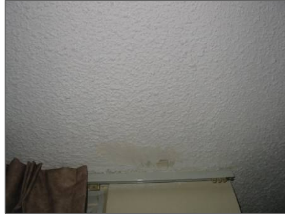
Texture coat ceiling
