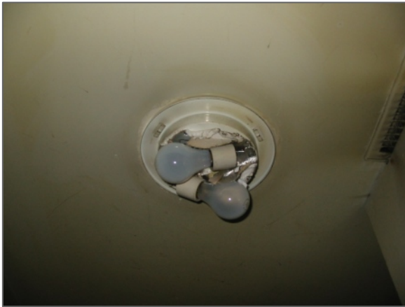
Paper heat shield on incandescent fixture
