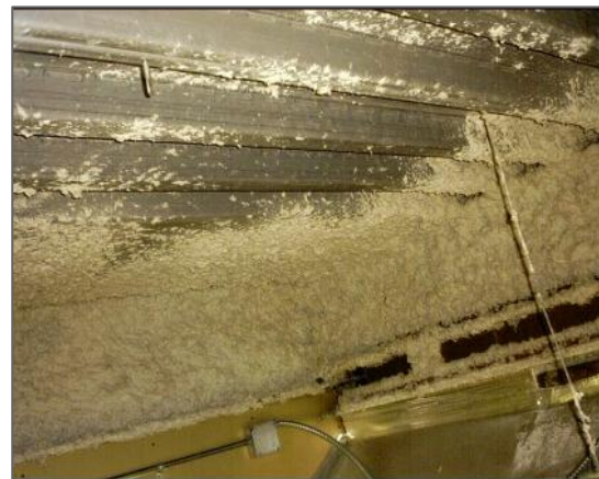
Fibrous sprayed fireproofing (beam only)
